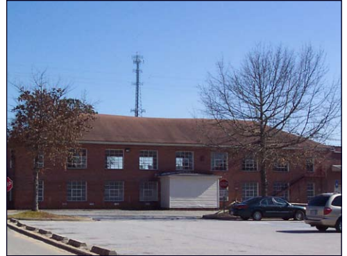
The R&R Building will be rehabilitated into a community arts building for local artists and residents.
