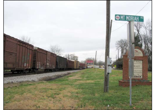
Mobility is limited with the railroad bisecting downtown. A new grade-separated crossing is needed in the near future to alleviate traffic issues.
