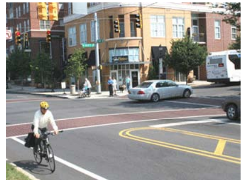
A "Complete Streets" approach to roadway design will help facilitate safer mobility in downtown.
