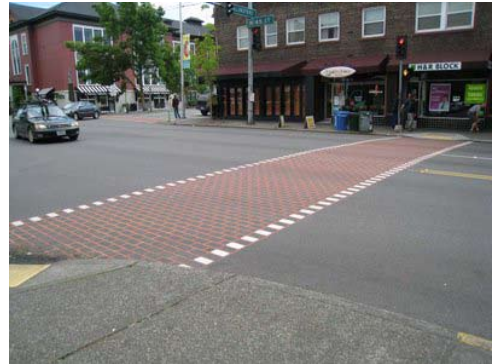
Crosswalks with textured paving will alert drivers that the roadway is to be shared with pedestrians.
