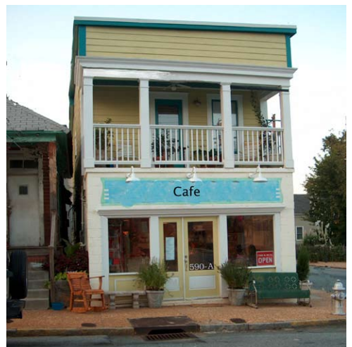
Rehabilitation of existing buildings will be most appropriate for retail and office use in the early development phases.
