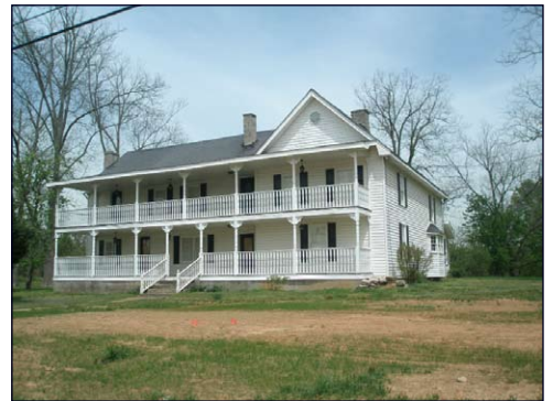
Downtown Auburn has a number of historic properties that are underutilized and could be rehabilitated for new adapted uses.
